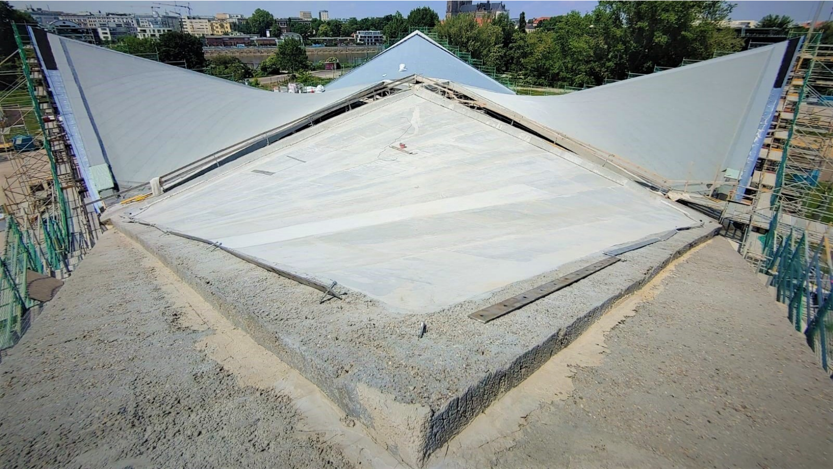
The hyparshell in Magdeburg after the application of the CARBOrefit® process. (©CARBOCON)
